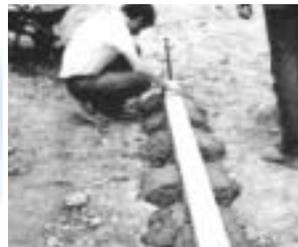
**3a.** The concrete bedding method\* requires a stiff concrete bedding slurry (somewhat dry) along the length of the trench. The bedding concrete should be as thick as the floor or driveway. Butt the channels together in the trench, on top of the concrete. Allow the concrete bedding to cover approximately 2" up the side of the channel. Align the top of the channel with the string line. Allow the concrete bedding to set. Connect the outlet piping as required.
